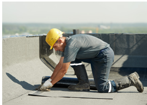
Roofing Contractor - NYC
